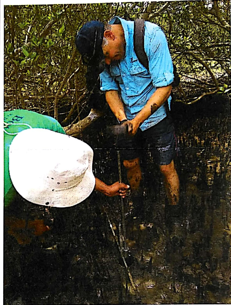
SAEON members install the rods for a benchmark within the mangroves at Nahoon.
